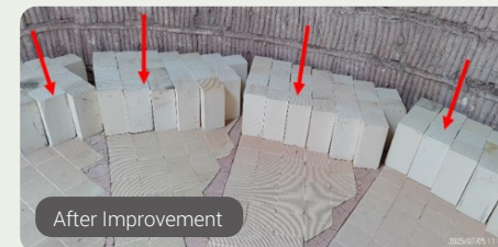
The installation of additional heat storage ceramic media increased heat storage capacity and heat exchange efficiency, reducing exhaust heat loss.
