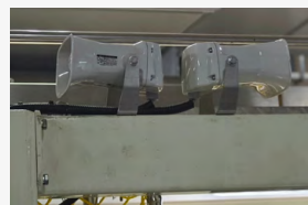
Zhongshan Site 70 Voice Reminder Units Added to the Automated Line
