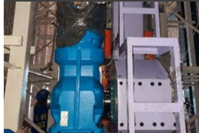
Explosion-proof motors in the general chemical warehouse were upgraded
